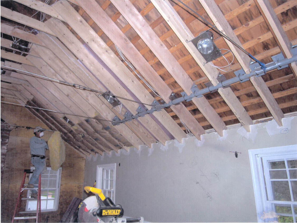
Figure 2 Cable Stayed Cathedral Ceiling Installation in Progress – Typical Both Sides
